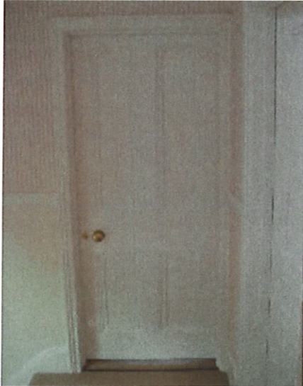
An original first floor bedroom door
