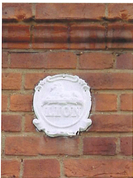
Detail of original brickwork showing Flemish bond and recessed pointing. The Lion badge was a plaque that certified that the house owner was subscribed to a fire insurance scheme.
