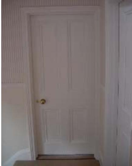
An original first floor bedroom door
